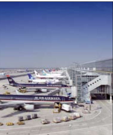
Lotnisko, Frankfurt Airport, Frankfurt
